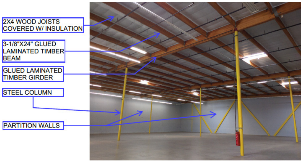
Figure 1: Existing Roof Structure on Stage B
